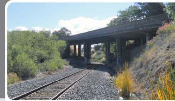
Active BNSF Railroad New bridge must meet clearance criteria and accommodate second track and access road.
